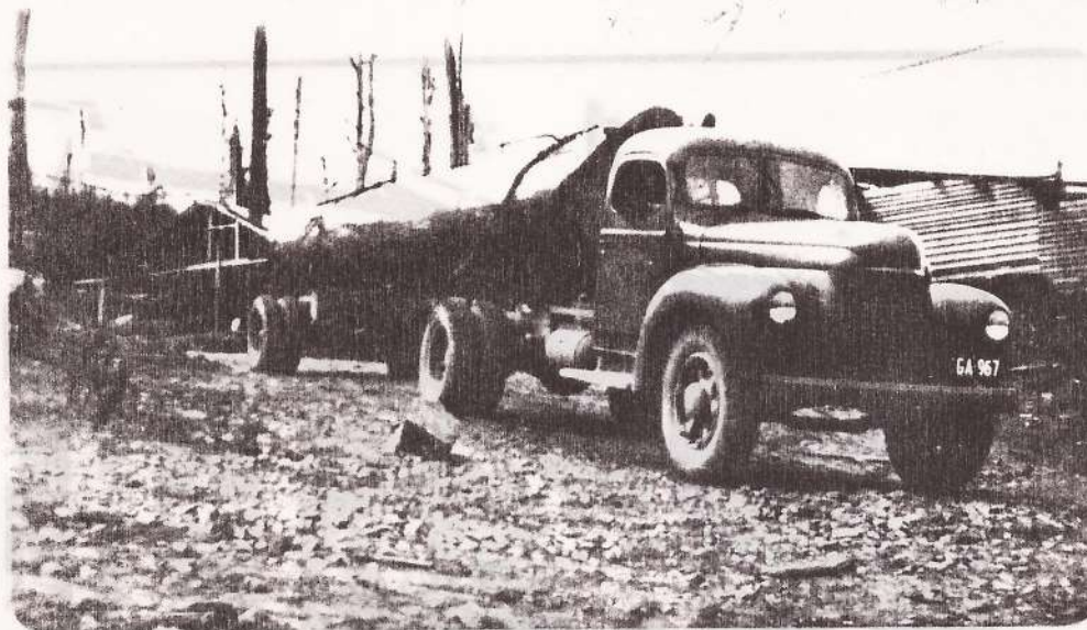
The old and new ways of carting timber from the Neulyn Mill. Above shows the tramway incline before the gantry was installed; the lower view shows the cartage of logs by road direct from the mill.
