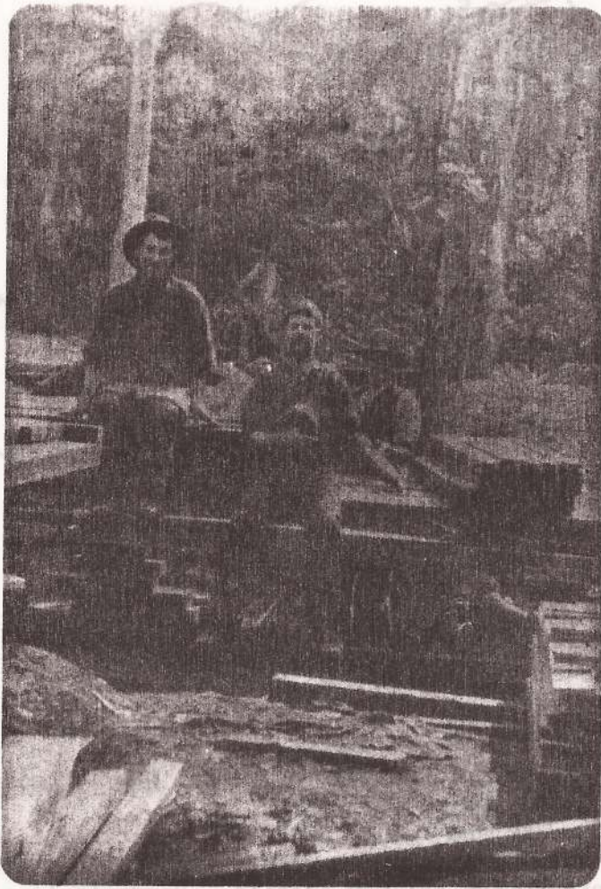
Some of our men at the loading dock, Mackie Creek. The timber is supported on blocks which were knocked away to lower the load onto the tram trucks.
