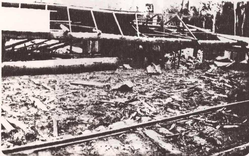
Installing the Mount Cowley mill after the flood.
